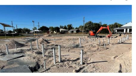
Construction on the Youth Centre has resumed, with the under-slab plumbing now finished. Next week, preparations will begin for the pouring of the floor slab, which is anticipated to be finished by mid-August.
