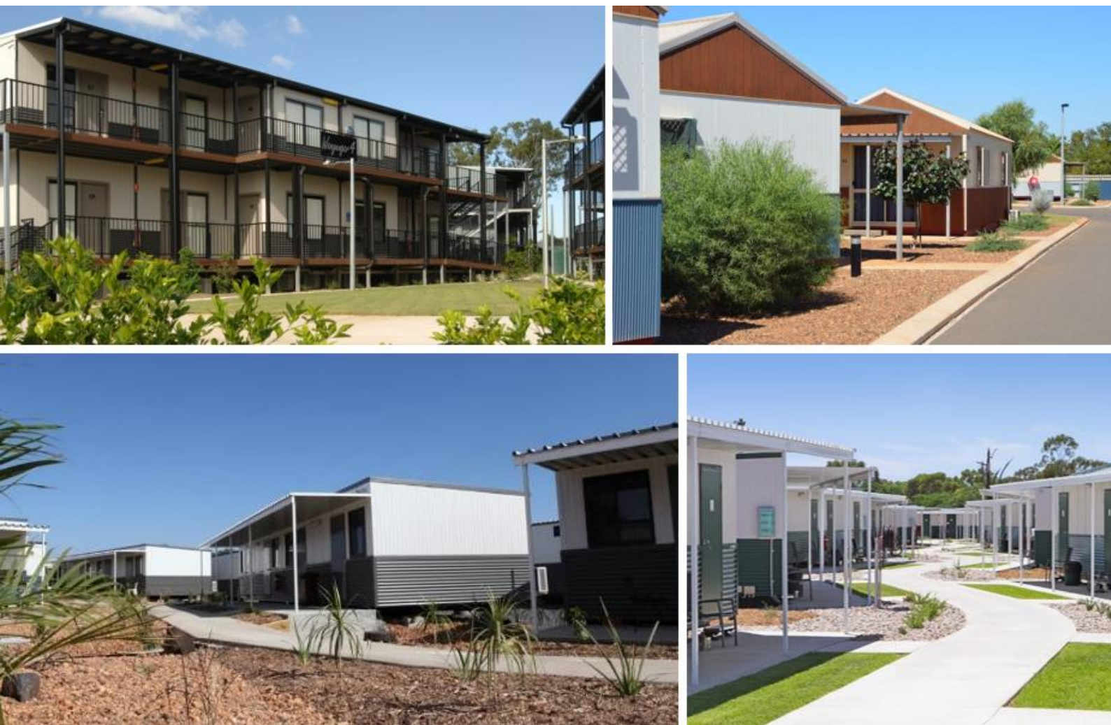
Figure 8: Long-Term Prefab Accommodation Precedents 2
