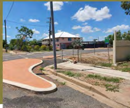
Image 8: Kerb ramp on the corner of Elderslie Street and Manuka Street
