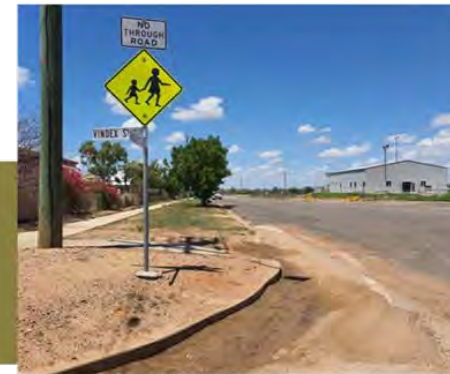
Image 7: Kerb ramp on the corner of Vindex Street and Fraser Street
