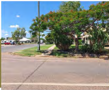
Image 5: Kerb ramp on the corner of Dagworth Street and Manuka Street
