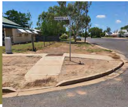
Image 6: Kerb ramp on the corner of Oondooroo Street and Vindex Street
