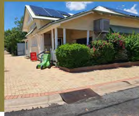
Image 9: Kerb ramp on the corner of Elderslie Street and Oondooroo Street
