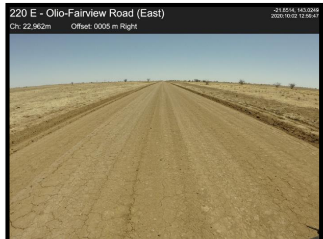
Flood Damage Works on Olio- Fairview Road
