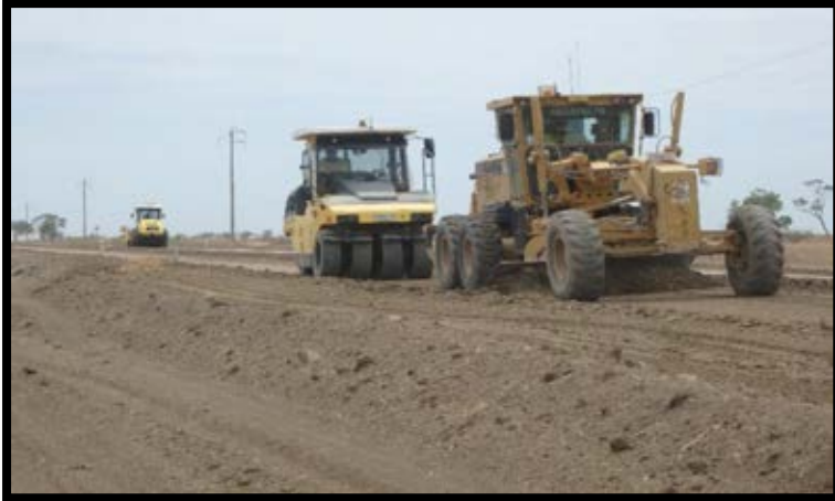
Hughenden Road Subgrade Works
